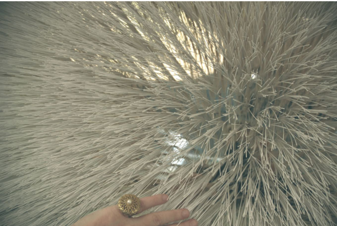
Inside Outside, Acoustic wall treatment for Mercedes Benz Museum, Stuttgart, Germany, 2006 (Architect: UN Studio) Detail of brush panel for the acoustic treatment of a curved wall in the coffee shop. The long, thin hairs are inserted within wooden panels clad with reflective metal, creating the effect of continuous (borderless) space.
